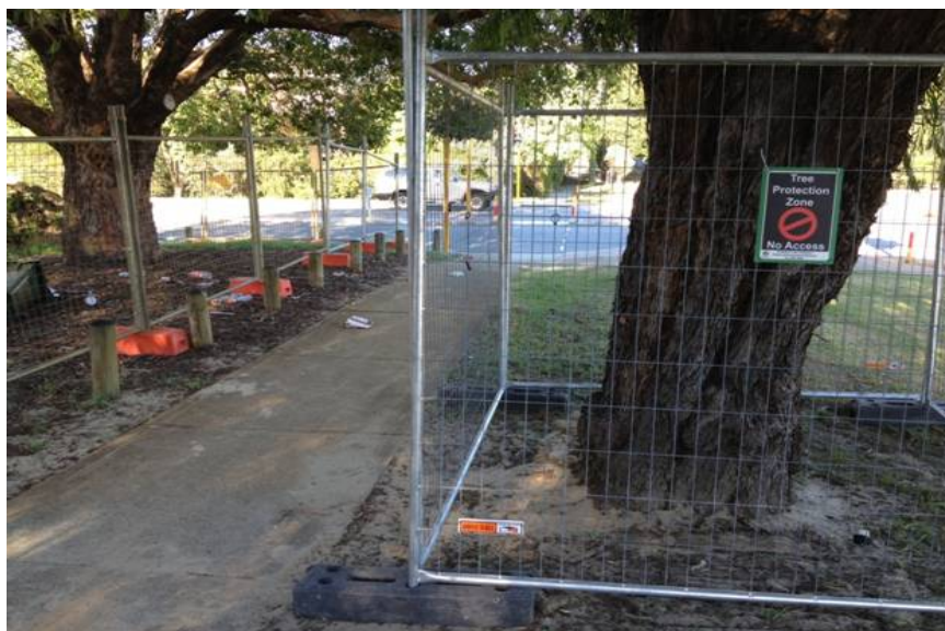
Typical Verge street tree protection barricade/fencing - with signage.
