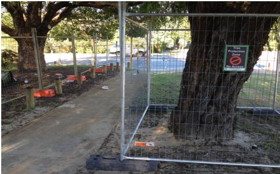
Typical Verge street tree protection barricade/fencing - with signage.
