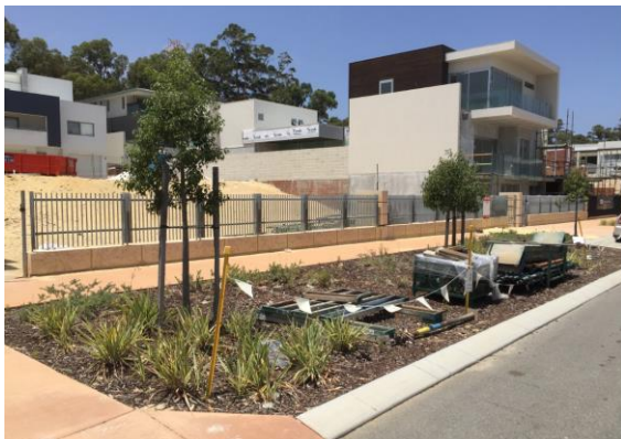
Building material placed on top of vegetation
