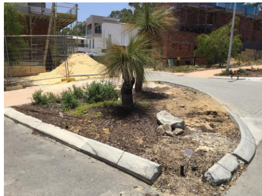
Damaged kerbing/sprinklers/plants by trucks
