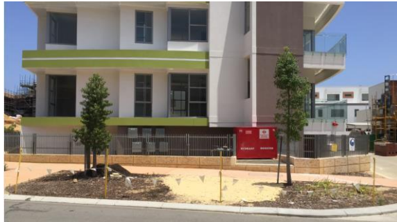
Site where building works are complete and verge landscaping can be reinstated by owner
