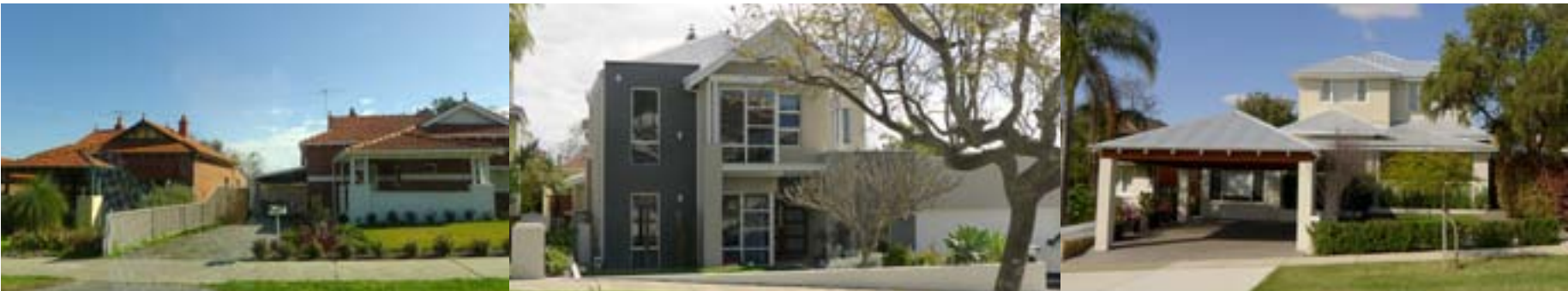
Rich roof forms of single storey Wembley homes do not necessarily translate
