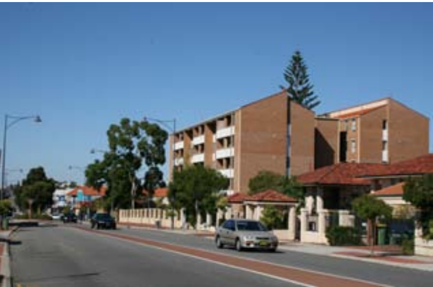
Existing tall buildings, although not necessarily beautiful, assist in orientation and way-finding in the town centre.
