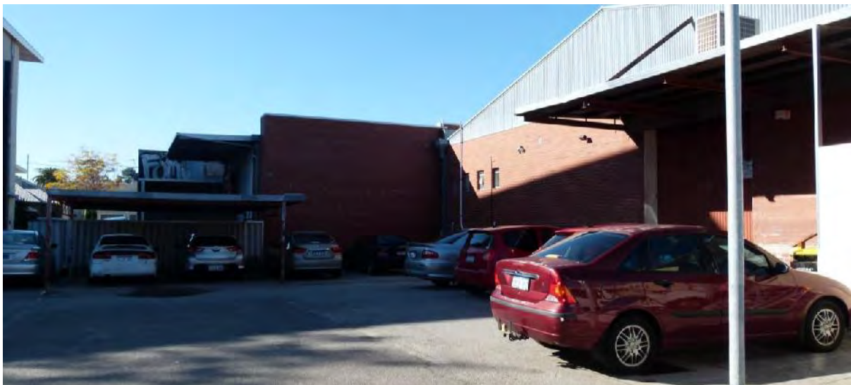
Photo 5 – Rear of the subject site viewed from Hull Lane.
