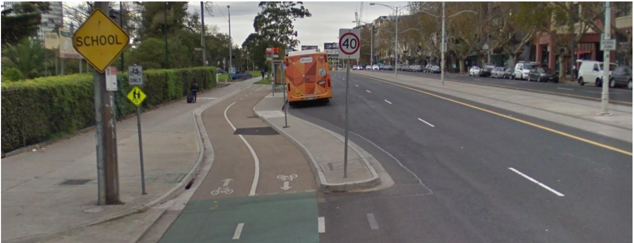
Figure 5-8 Protected/Separated Bidirectional Cycle Lanes, Solid Kerb Separated – Fitzroy Street, St. Kilda VIC
