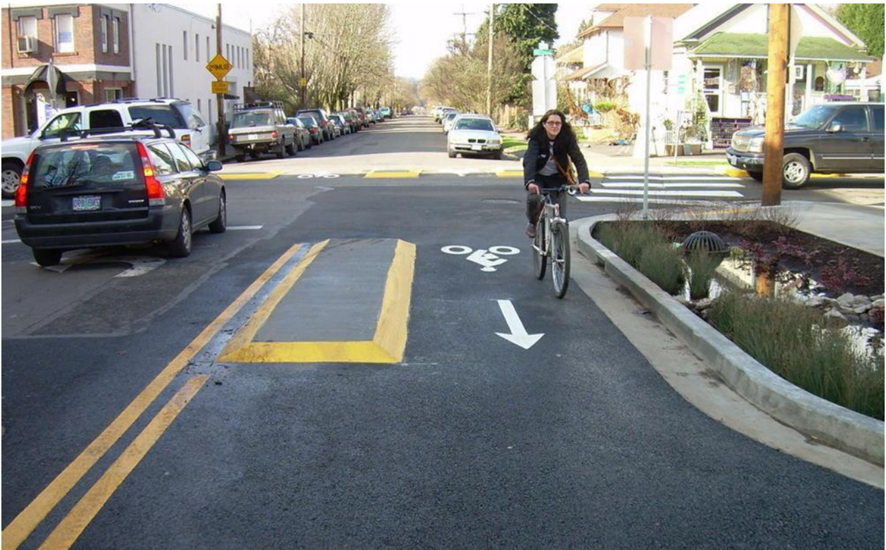
Figure 5-4 Spokane Street Bicycle Boulevard Utilising Contra-Flow Bicycle Lane with Partial Road Closure – Portland, Oregon USA
