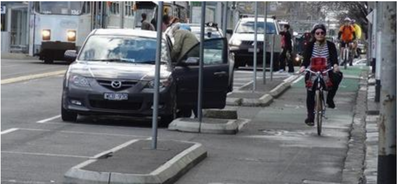
Figure 5-6 Protected/Separated One-way Cycle Lanes, Between Parked Cars and Road Kerb – Swanston Street, Carlton VIC
