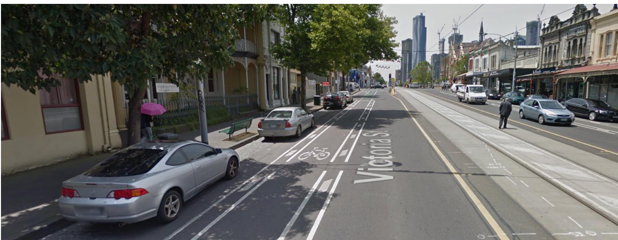
Figure 5-7 Protected/Separated One-way Cycle Lanes, Painted Chevron – Victoria Street, North Melbourne VIC
