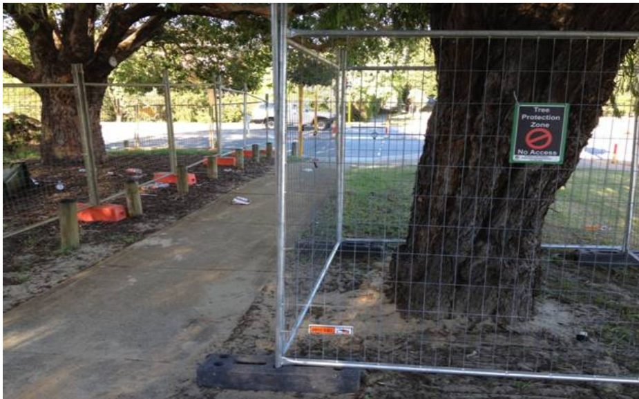
Typical Verge street tree protection barricade/fencing - with signage.
