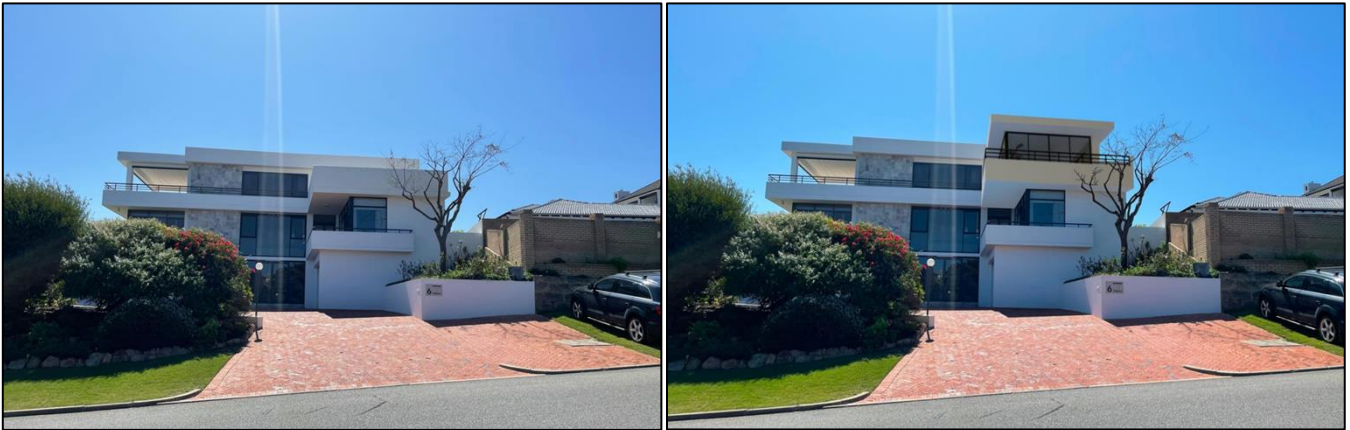
Figure 34: Left image: Photo of the existing dwelling as view from Yaltara Road. Right image: Site photo of the existing dwelling with the proposed third-storey extension superimposed.
