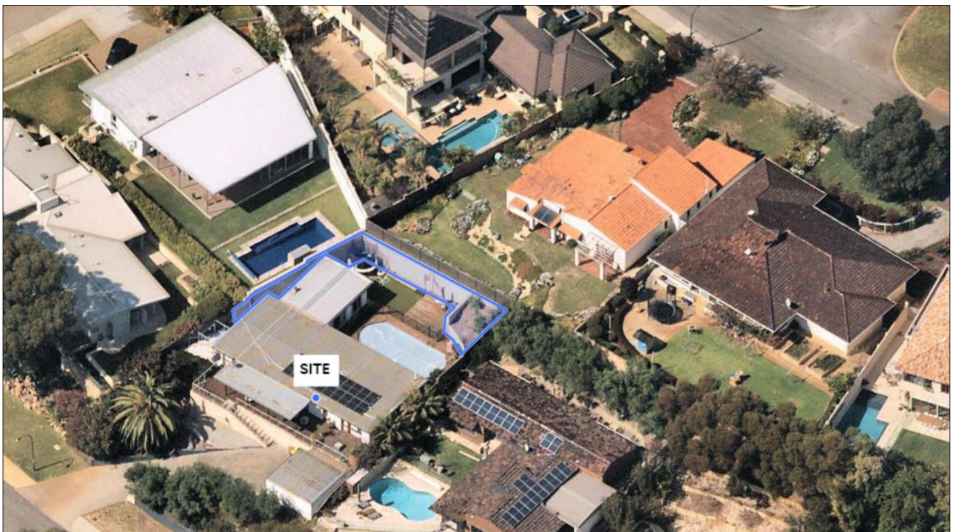
Figure 4: Nearmaps panoramic image showing the location of the existing large retaining walls (blue outline) at the rear of the subject site.
