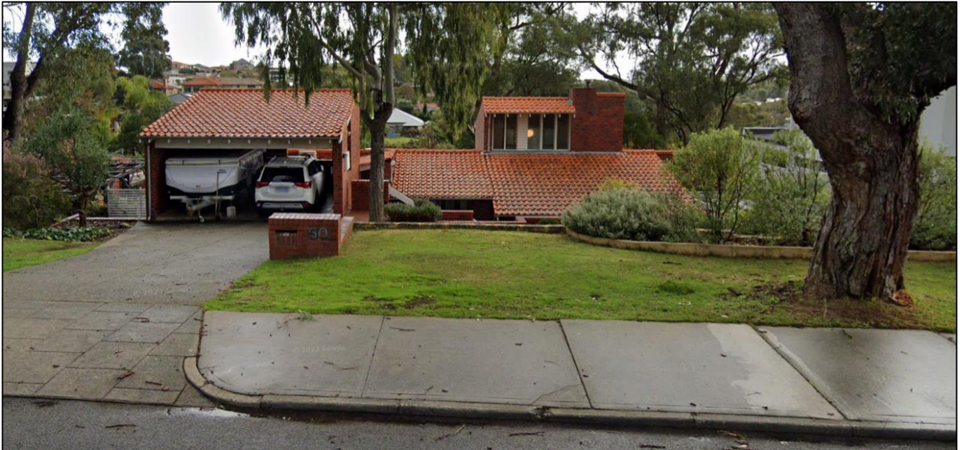
Figure 1: Google Streetview image showing the existing carport level is just below the street level and the existing dwelling sits significantly below the carport.
