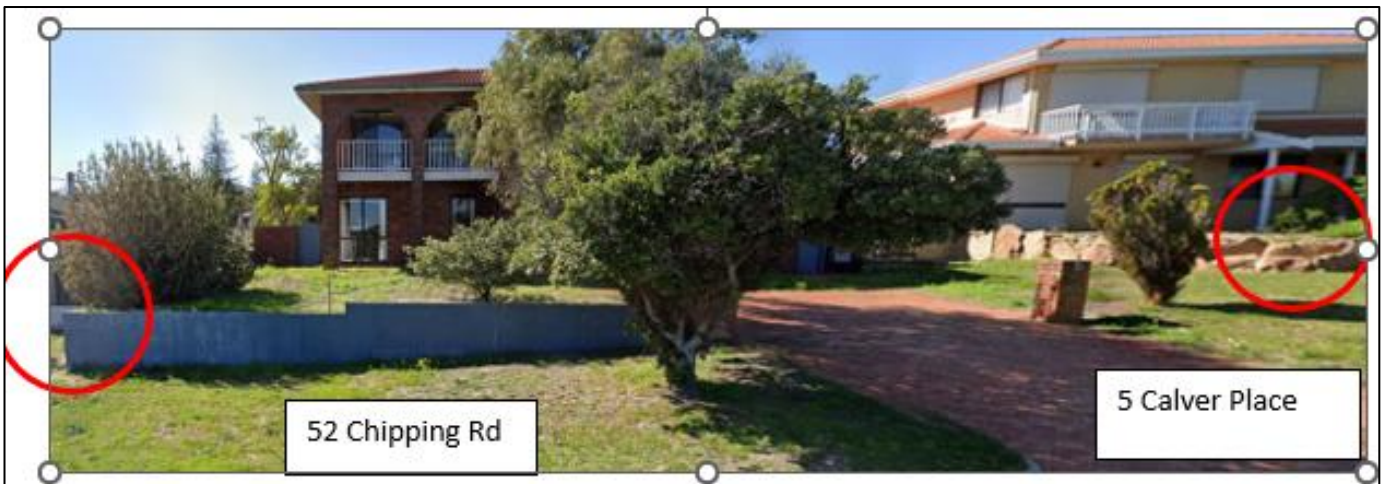
Figure 30: Neighbouring retaining walls within the front setback.
