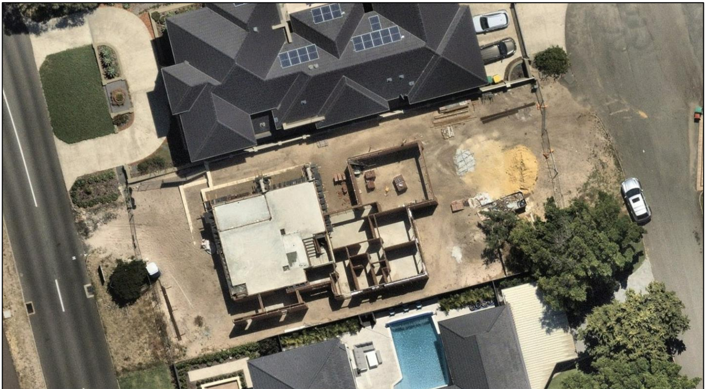
Figure 28: Nearmaps aerial image showing the extent of construction works already carried out on the site.
