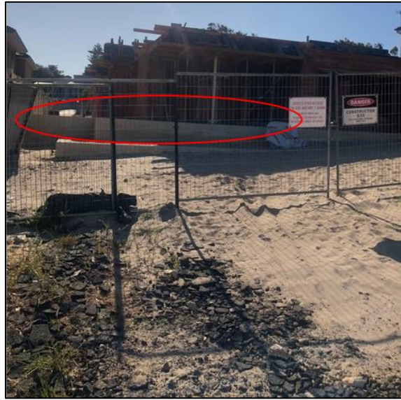
Figure 31: Subject retaining wall built 5m from front boundary
