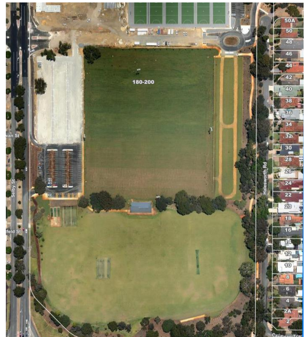
Carpark construction - January 2014
