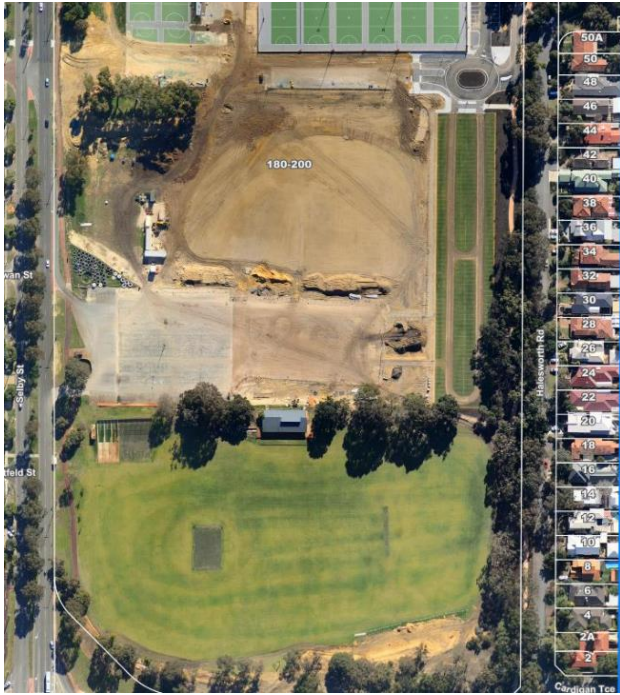
During construction - June 2013
