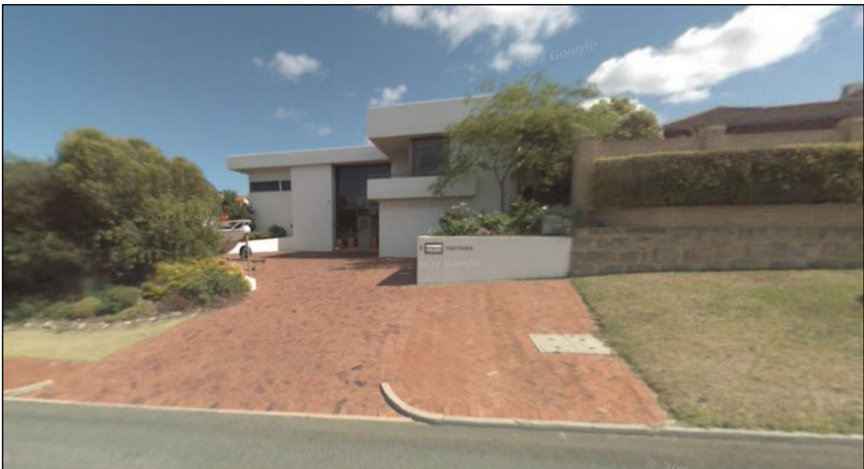
Figure 2: Google Streetview image dated December 2007 showing the existing dwelling was two-storeys from Yaltara Road.
