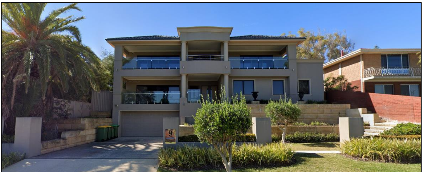
Figure 223: Google Streetview image of 9 Talgarth Way, which presents as three storeys to the street.
