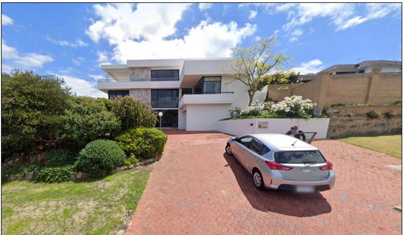
Figure 4: Google Streetview image dated October 2019 showing the existing dwelling is three storeys from Yaltara Road.
