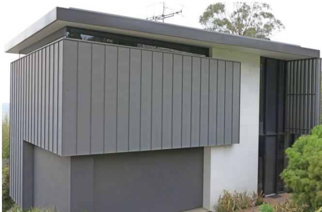
Figures 1 & 2: Copper weathering chart (top) and Zinc Quartz cladding (bottom).
