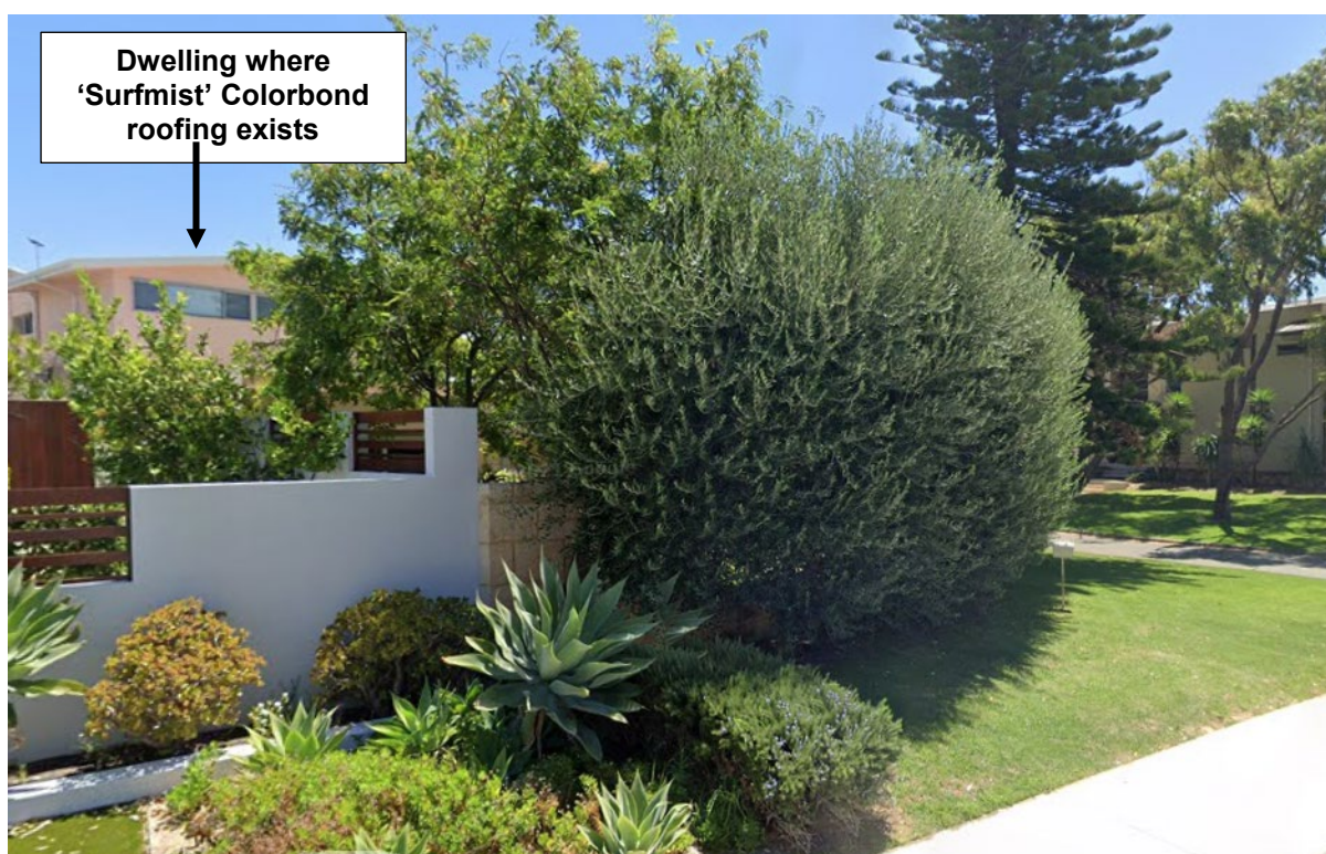
Figure 4 – View of the roofing from Branksome Gardens
