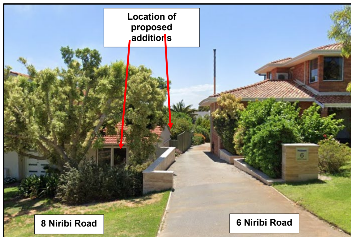
Figure 6 – Photograph showing the difference in ground level between 6 and 8 Niribi Road
