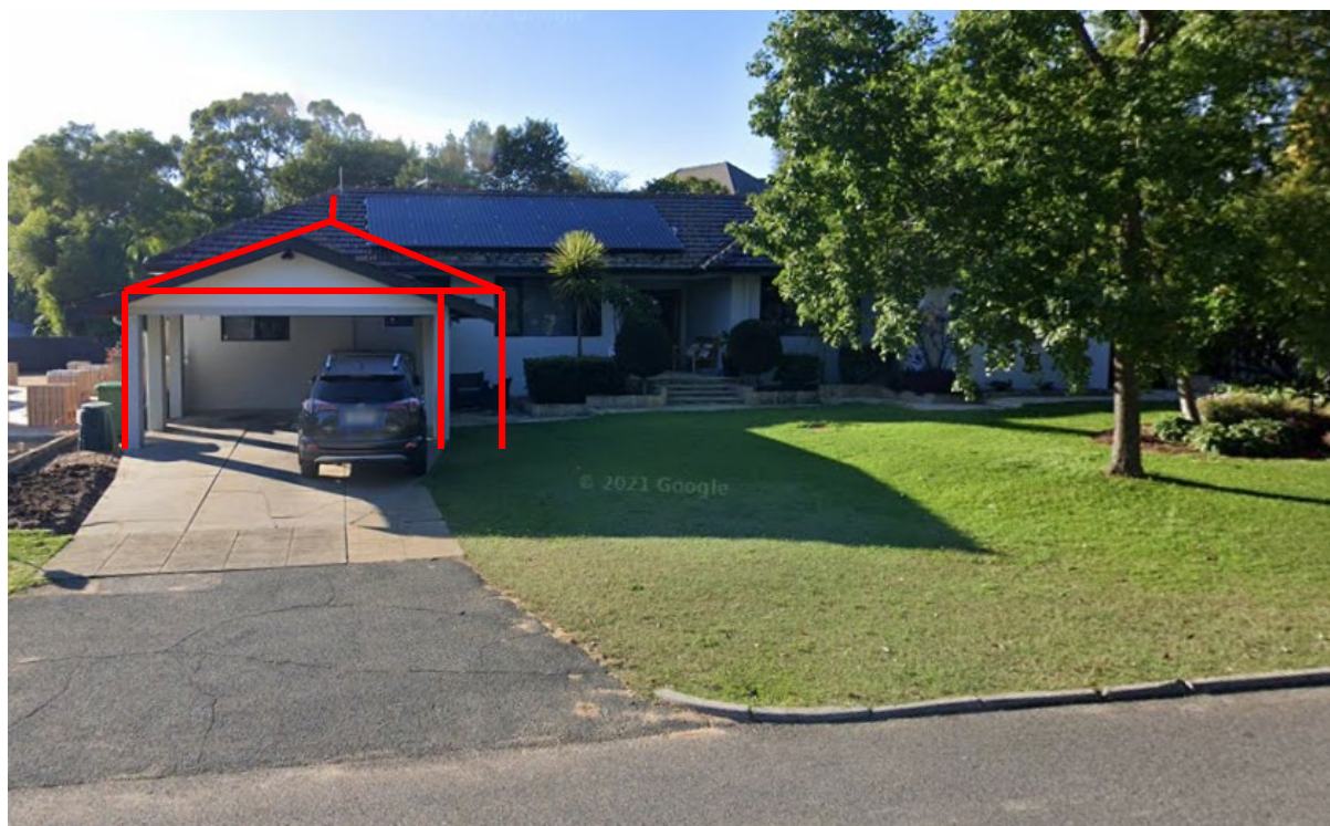
Figure 3 – Subject site as viewed directly from Tralee Road.
