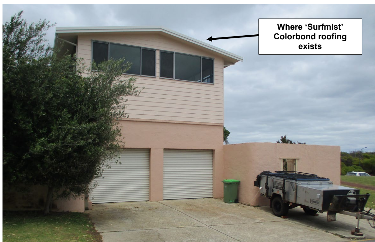
Figure 5 – View of the roofing from Dartmouth Avenue
